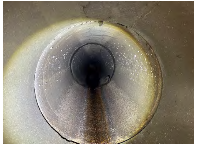
Inside culvert exit
