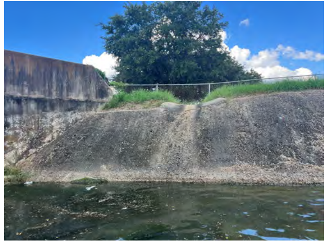
Facing out from culvert exit
