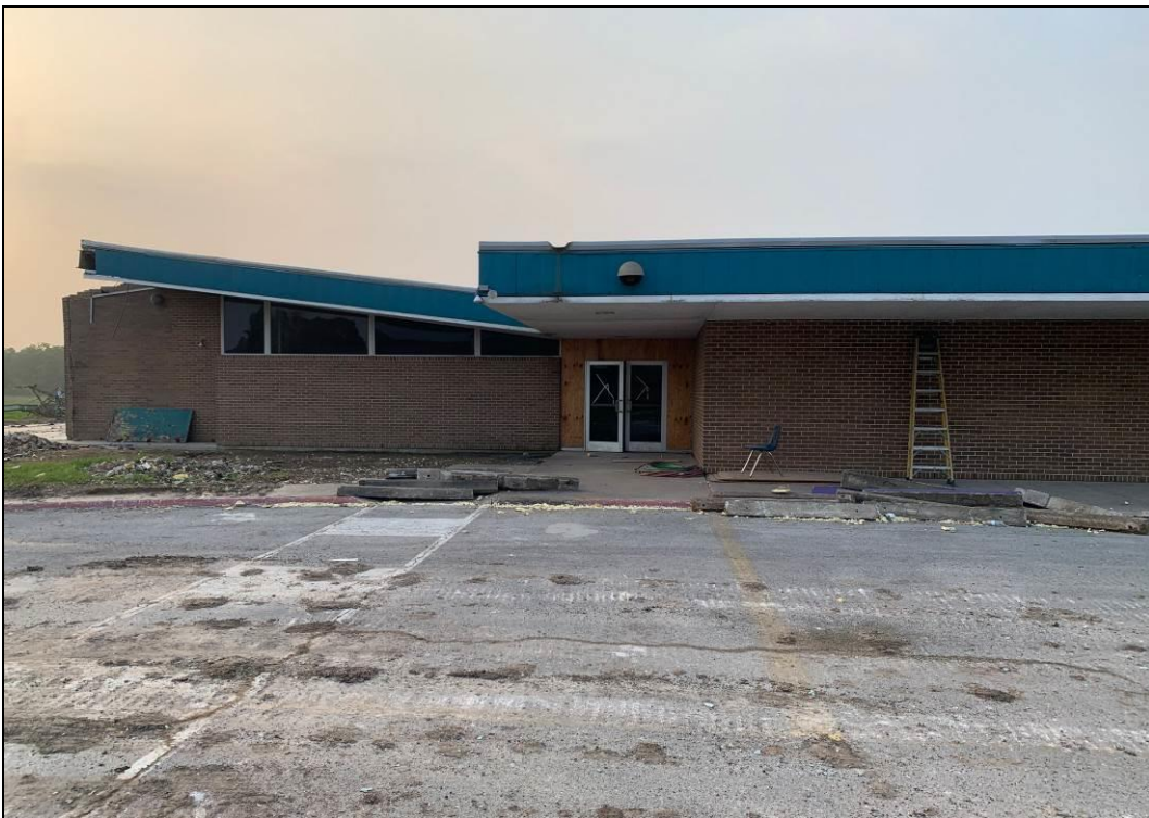
Figure 2: View of the school, facing southeast
