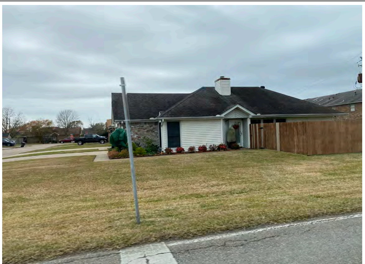
Typical view of structures in the Benefit Area.
