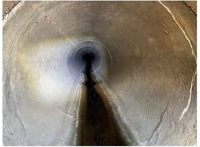
Inside culvert exit
