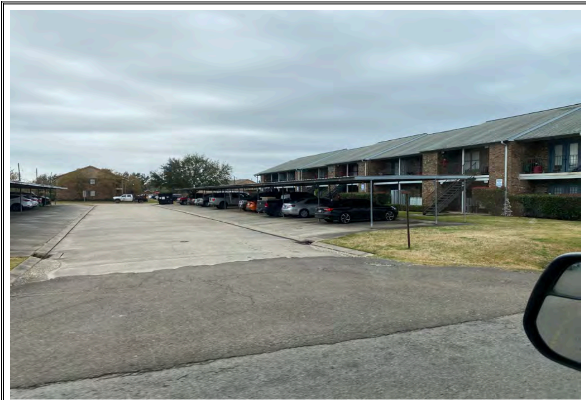
Typical view of structures in the Benefit Area.
