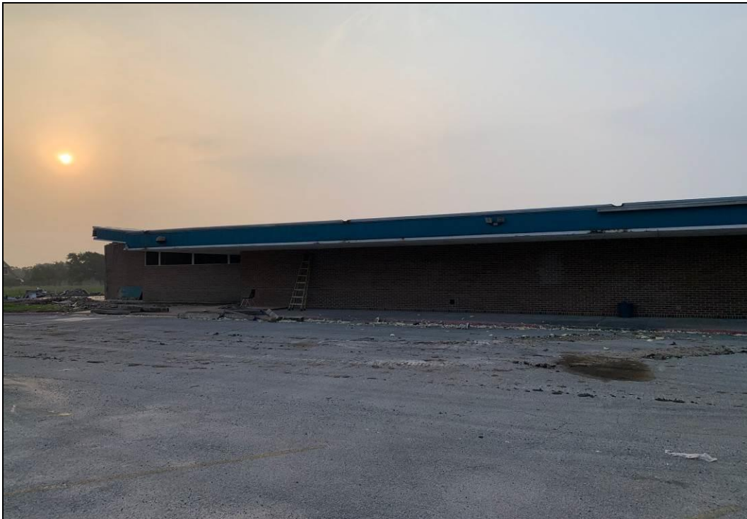
Figure 4: View of the school facing southwest
