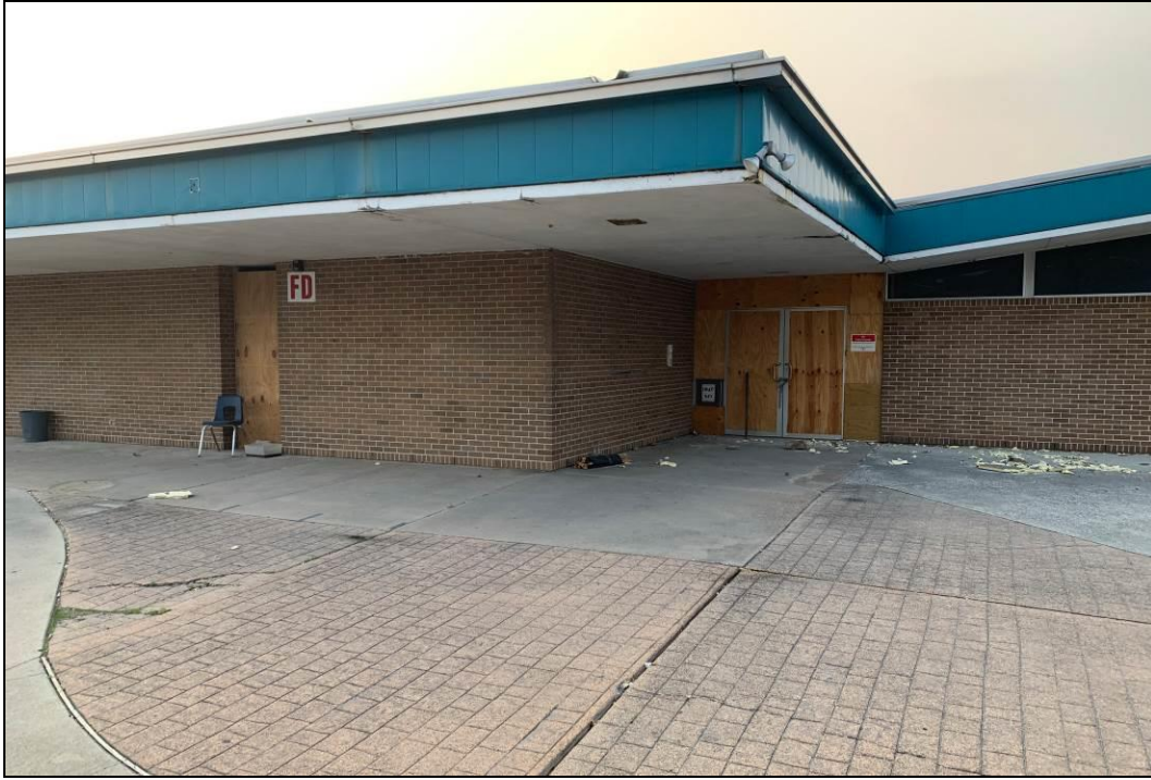
Figure 5: View of the school facing southeast
