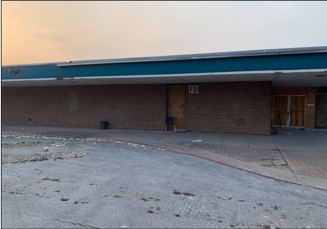
Figure 3: View of the school facing southeast
