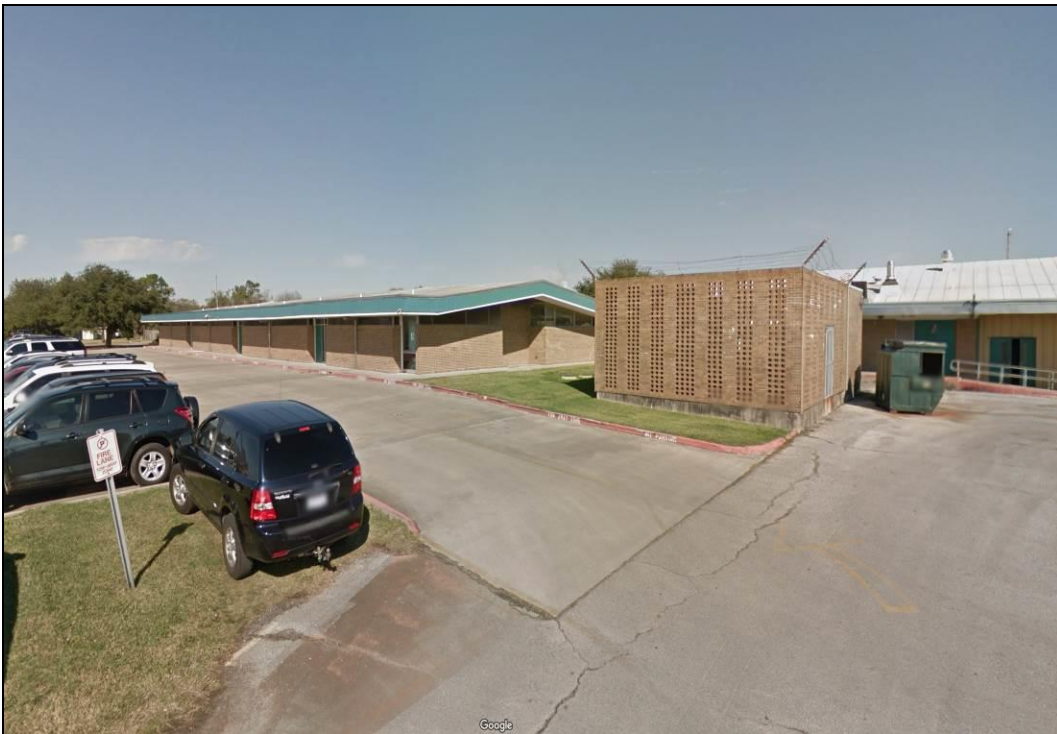
Figure 6: View of the school and addition, facing north
