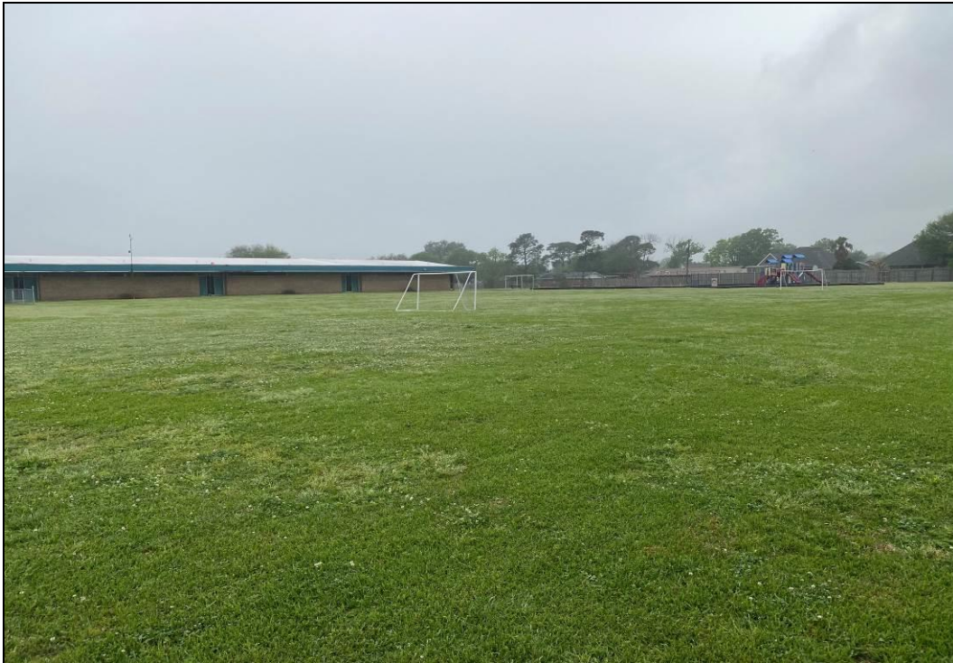
Figure 7: View of the school facing southwest
